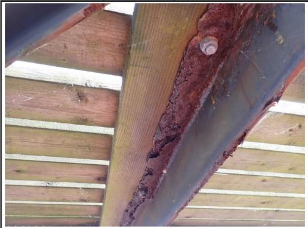
Photo 26: LOS to bay 2 cross beam, span 12
