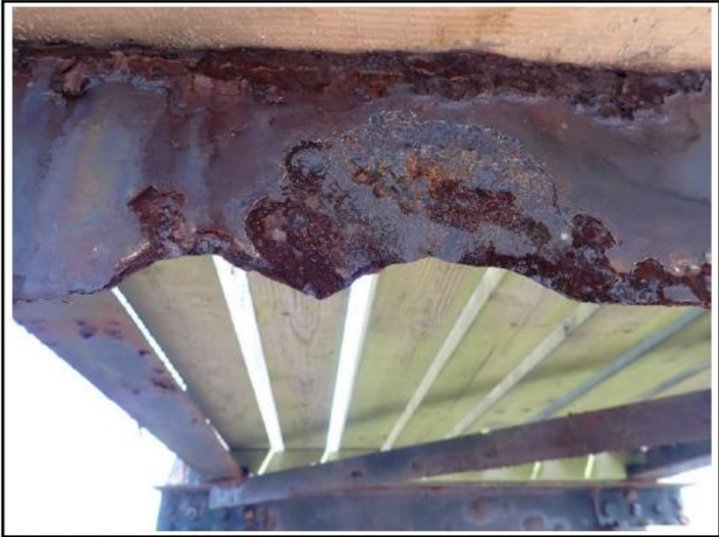
Photo 25: LOS to bay 9 cross beam Span 10
