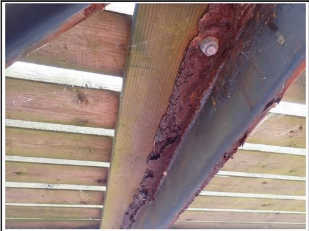
Photo 26: LOS to bay 2 cross beam, span 12
